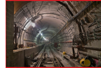
MTA Independent Engineering Services, New York, NY
