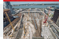
Hudson River Tunnel Replacement (Gateway Project), New York, NY
